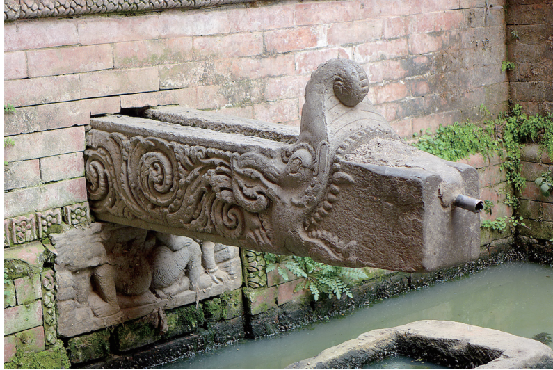
Fig. 3 Water spout, Licchavi period (apart from the metal spout fixed by cement).
